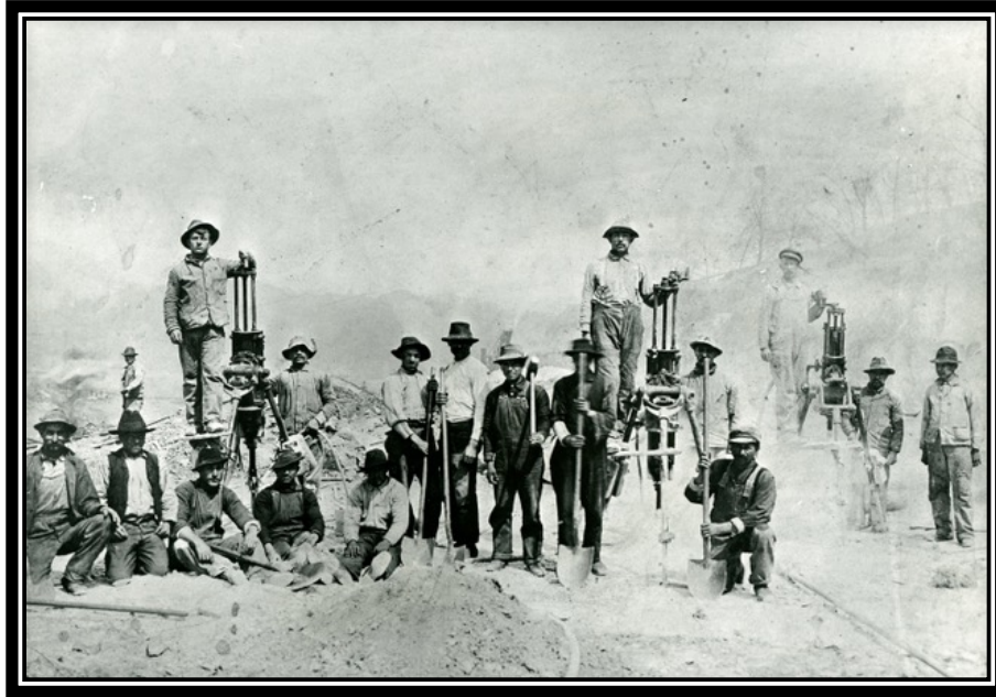
A group of Cornwall Ore Bank Company Workers, circa 1915, pose with two-man drills and shovels. One drill could do the work of 12-14 men.
